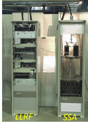
2001 – Booster 900 W @ 476 MHz ELETTRA Cavity
