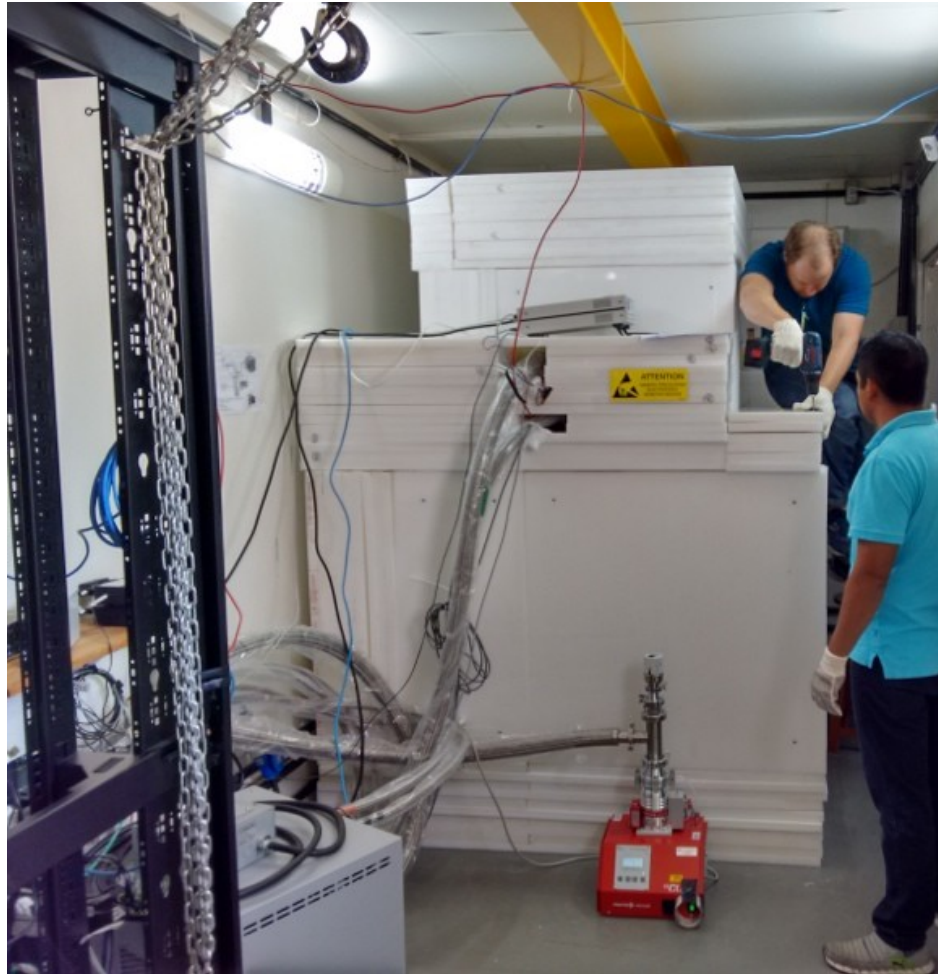
Finishing the shield
