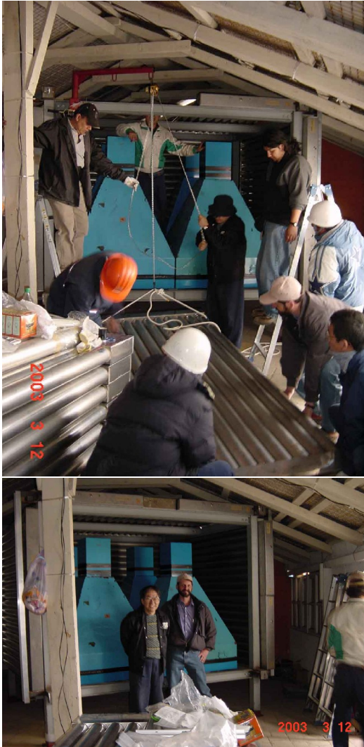
Fig. 9. Solar neutron telescope under construction at Sierra Negra on March 12, 2003.
