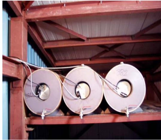
Figure 3: Front panel of the first module of the neutron flux meter at BEO Moussala
