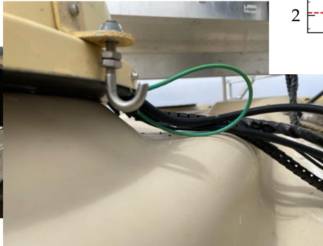
Figure 3: Grounding cable loop in The Nameless PhD
