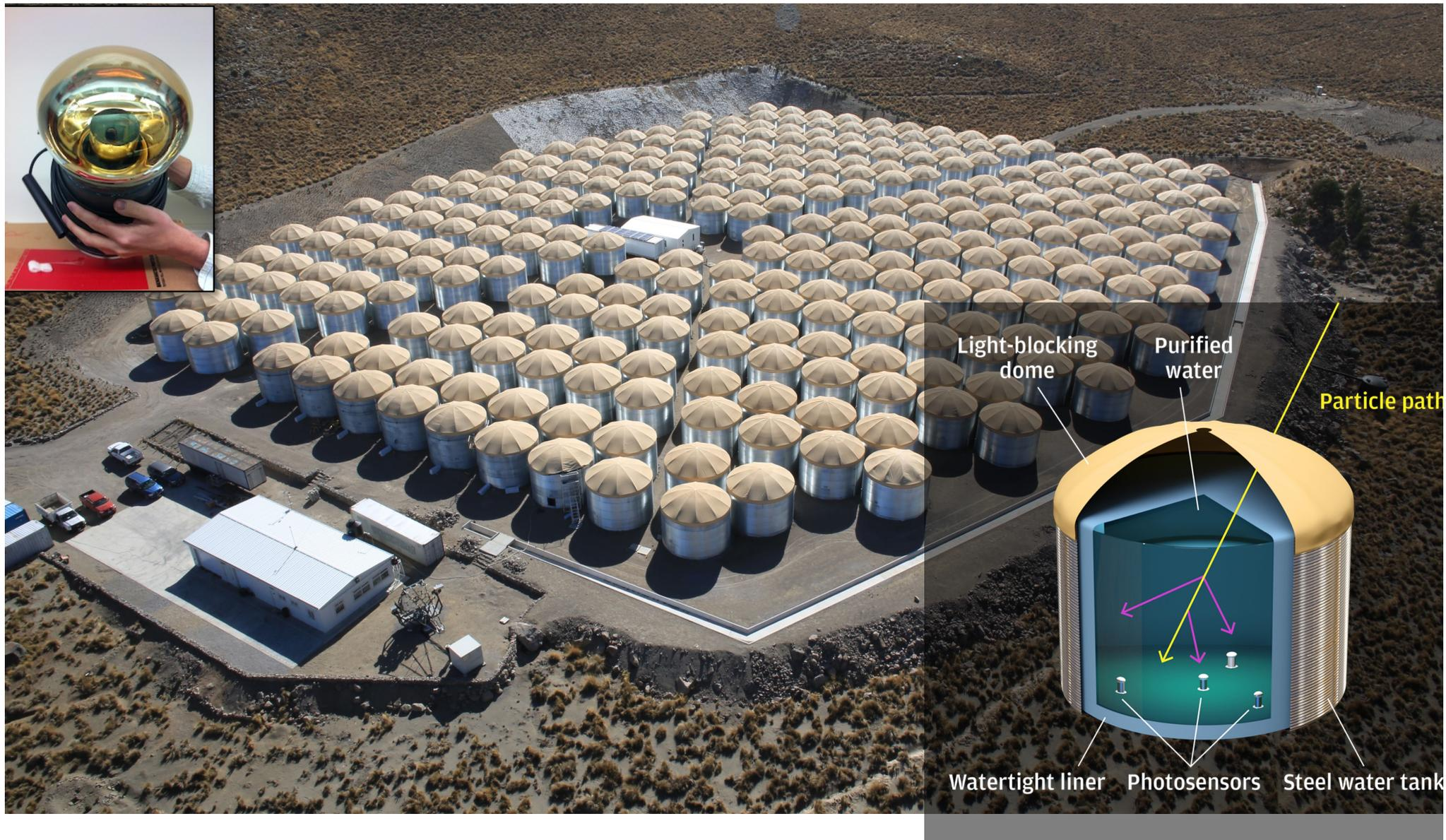
300 close-packed optically isolated water Cherenkov detectors
